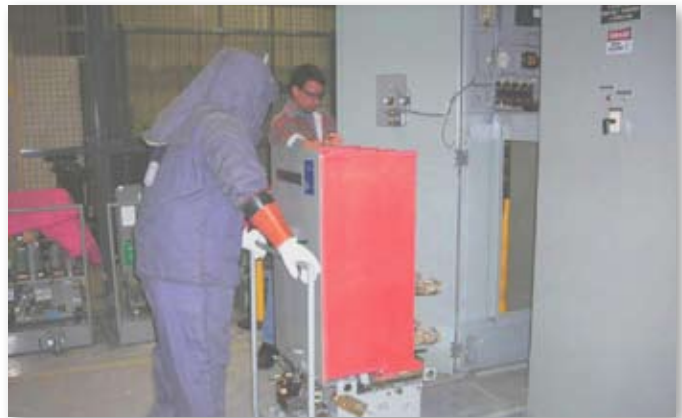
Instruction on installation of high voltage circuit breaker.
