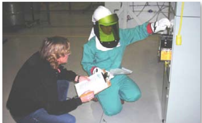
Job Performance Measure (JPM) testing on electrical equipment.
