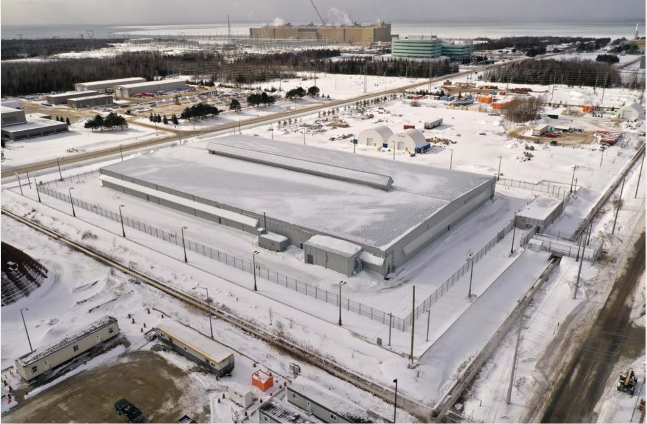
A new storage building was constructed in 2021 on the Bruce Site at OPG's Western facility to store used fuel from Bruce A and B.
