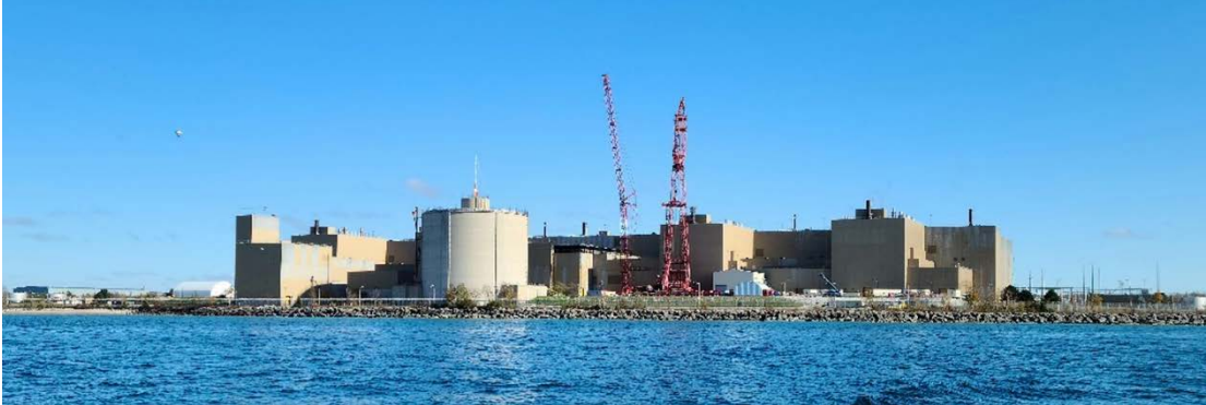
Figure 58 Cranes constructed in support of MCR at Unit 6
