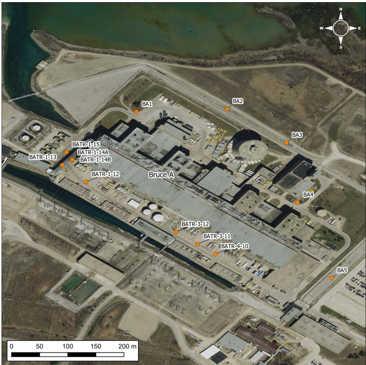
Figure 45 – Groundwater Monitoring Locations at Bruce A
