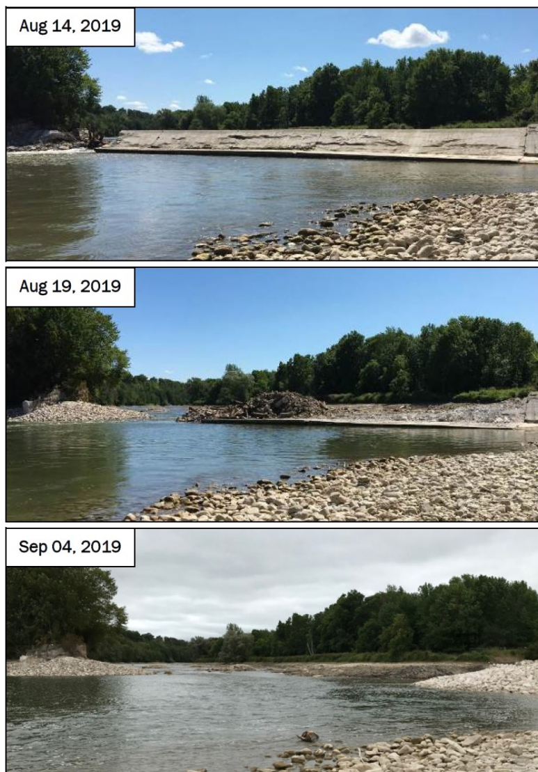
Figure 49 - Truax Dam, Walkerton, Ontario. The original wooden dam was built in 1852 and later replaced by the concrete structure shown above in 1919. The dam posed a significant barrier to fish passage for more than a century before it was removed in the summer of 2019 over the course of 3 weeks
