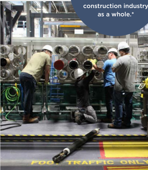
Millwrights and Boilermakers in a replica of the vault. For three weeks, they trained on the specialized tooling before moving to site for the first Major Component Replacement project of Unit 6 (MCR6).
